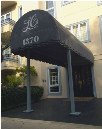
Figure 3: Building with a canopy that shades the entrance from direct sunlight. A darkened floor further reduces glare from sunlight.
