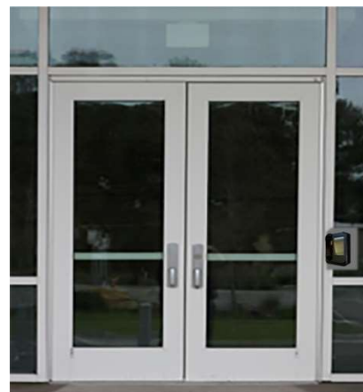
Figure 1: Doorway entrance with Access200w on right, angled to avoid sunlight. In this solution, the Access200w faces users making it convenient for them to look at the faceplate from a position directly in front of the entrance door. The darker colored mount also reduces glare.
